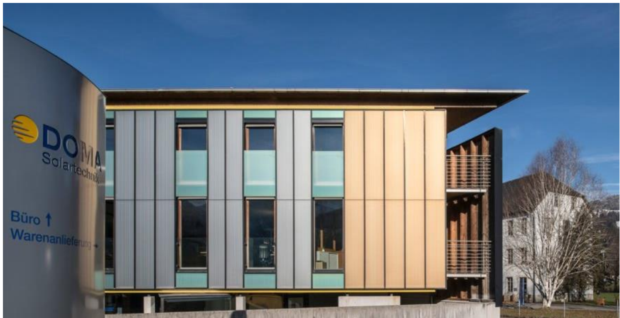
Fig. 5: elevation view showing façade integrated pv panels with colour on DOMA Solartechnik GmbH Headquarters building, Satteins, Austria [20]
